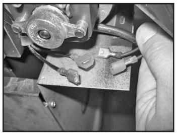
Figure 21: Disconnecting fan wires.
