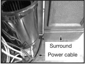
Figure 31: Routing power cable through the surround.
