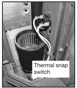
Figure 30: Re-attaching thermal snap switch.
