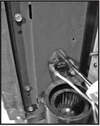
Figure 22: Unscrew thermal snap switch.
